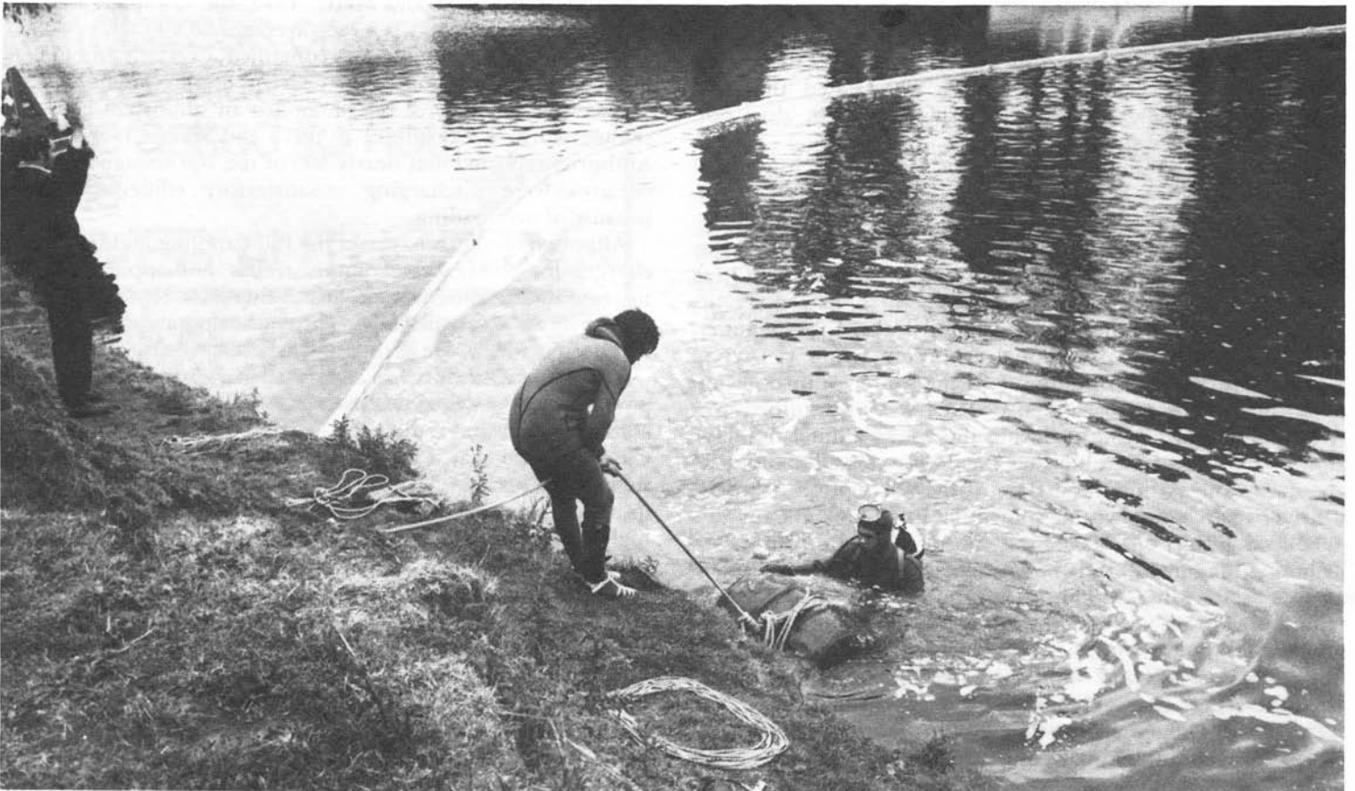
A boom laid by the Wessex Water Authority to contain oil and other pollutants
